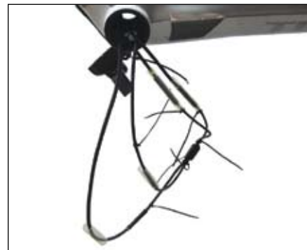
Figure 7. Anti-noise zip-ties on electric cables.
